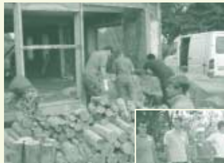
Above: The salvaged cordwood logs are reused
