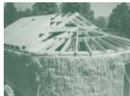
A Straw bale building by Amazon Nails
